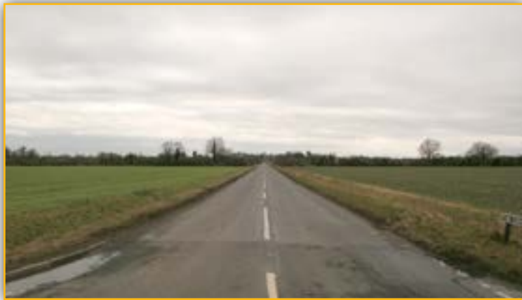
Your vision is naturally projected further ahead. Because of the absence of any foreground hazards
